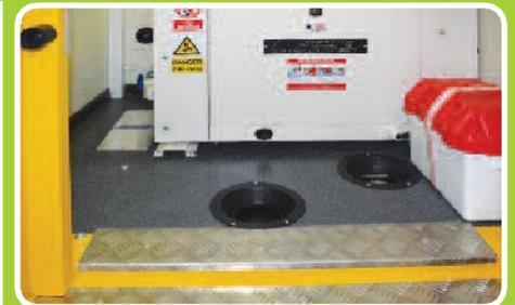
Anti-Slip floor used in a container
